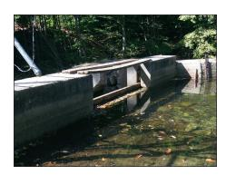
Our Pleasant Lake and Parker Pond dam has been totally rebuilt over the winter and is functioning flawlessly. With a spillway and a gate to control outflow, the historic lake water level will be easier to maintain for the next hundred years. An inch of lake water depth equals approximately 40 million gallons of water. The outflow capacity of the new structure
