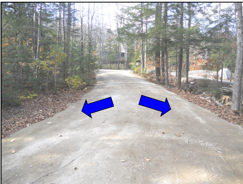
This driveway off of Heniger Park Road in Otisfield was recently built up, crowned and compacted to divert water into adjacent vegetation.
