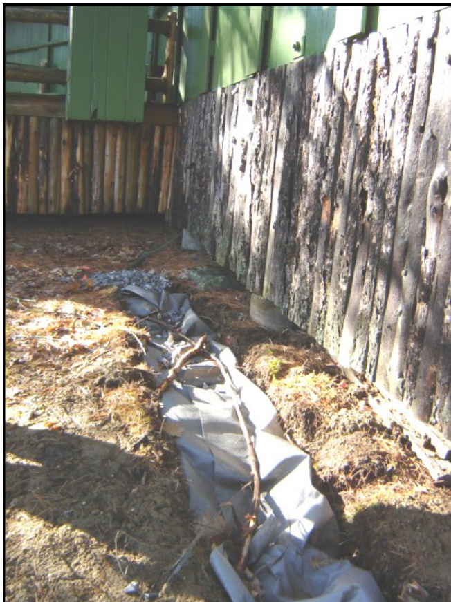
Drip line trenches being constructed along Camp Arcadia's cabins.
