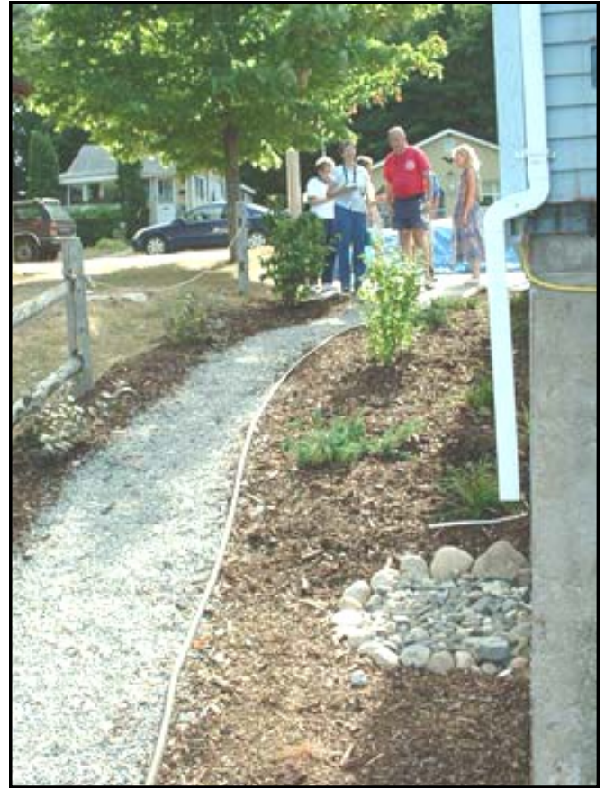
Drywells are deep reservoirs of stone used to infiltrate stormwater from roof gutter downspouts.
