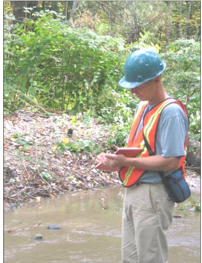
Chris Baldwin, CCSWCD Engineer, oversees work being done at a construction site.
