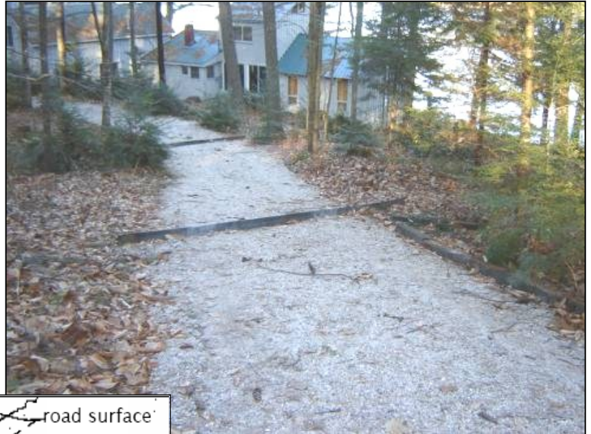
Pictured above is a series of rubber razor water diverters placed on a driveway in Denmark, Maine.
