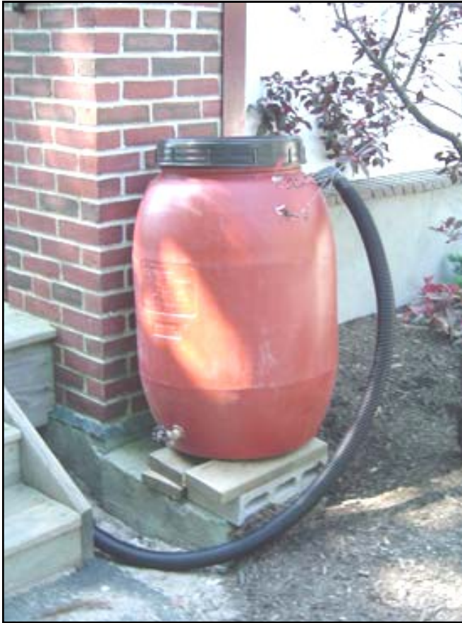
Rain barrels capture roof runoff from gutter downspouts to be used at a later time for activities such as watering gardens and flowerbeds.
