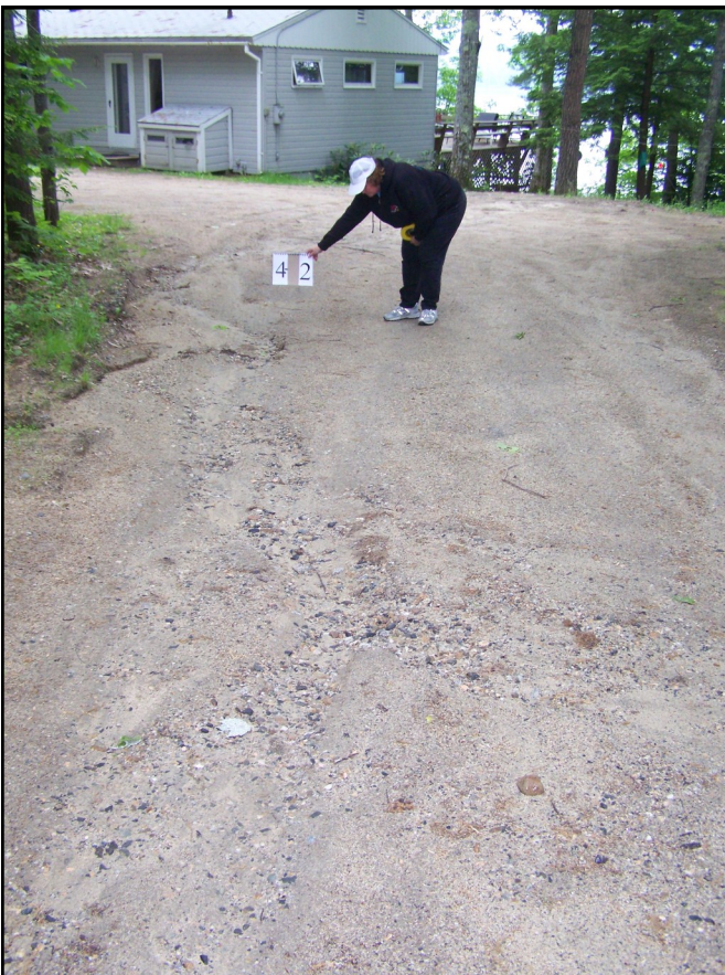
Site identified in the 2006 survey in which sediment is washing down a driveway and into Pleasant Lake.
