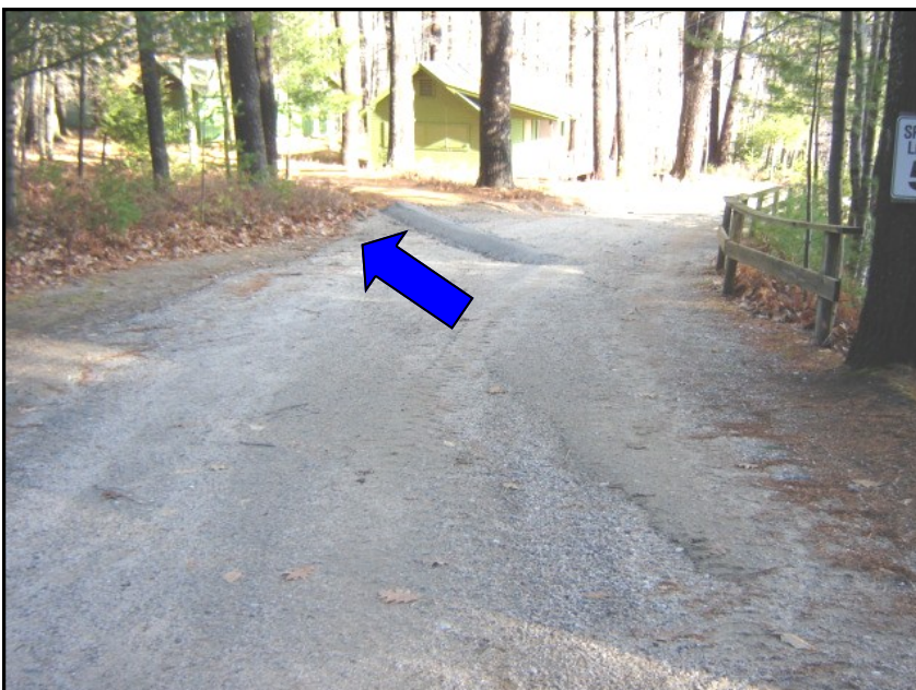
This "speed bump" water diverter was created at the top of a gravel road at Camp Arcadia to direct stormwater off the road into stable vegetation.
