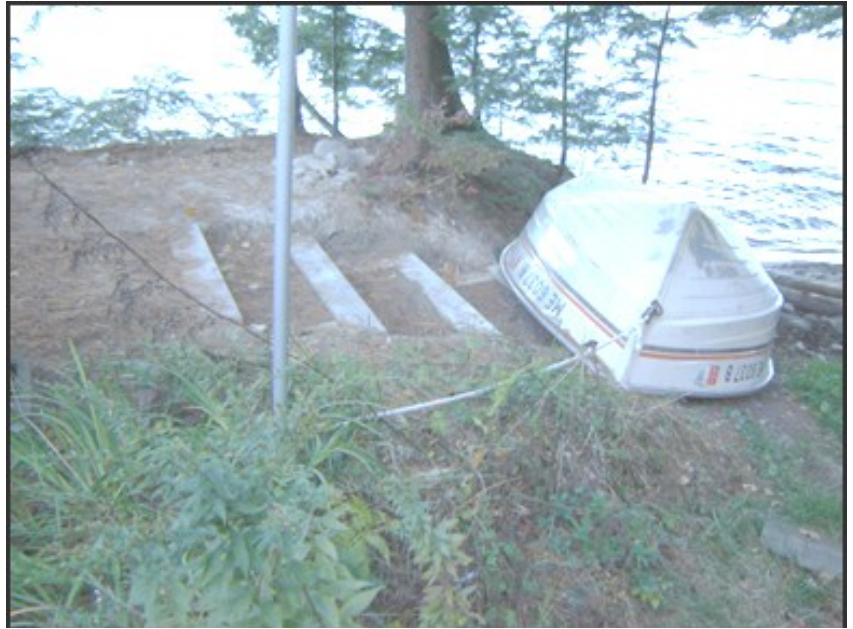
Infiltration steps leading to Pleasant Lake's shoreline were created at this residential site off of Scribner Lane in Casco..
