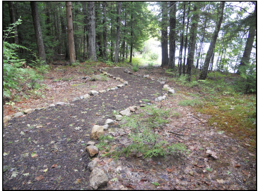
Above is a meandering pathway at Camp Arcadia in Otisfield leading to the shoreline of Pleasant Lake. Erosion control mulch, stones, and native plants were used to direct foot traffic.
